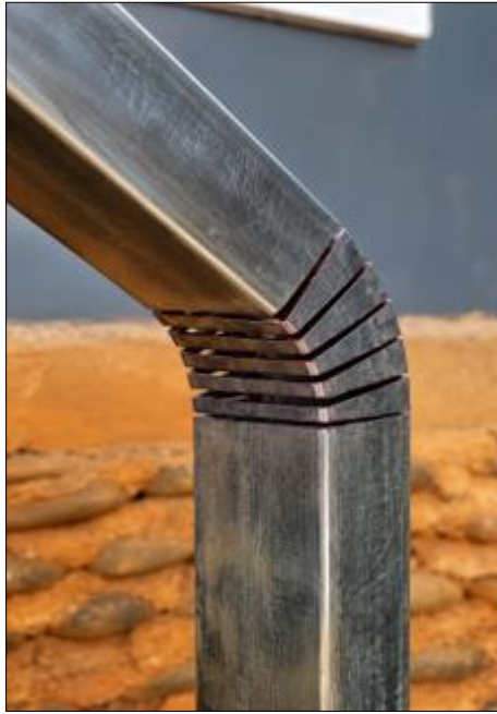
Fig 8: Wider view of the same segmented bend, showing the transition from the curved handrail section into the straight vertical post.
