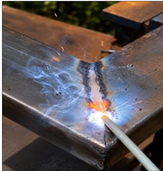
Fig 6: Shielded metal arc welding in progress at a mitre corner joint of mild steel plate.
